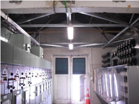
Figure 5-15 Seismic Strengthening at Adelaide Road Substation
