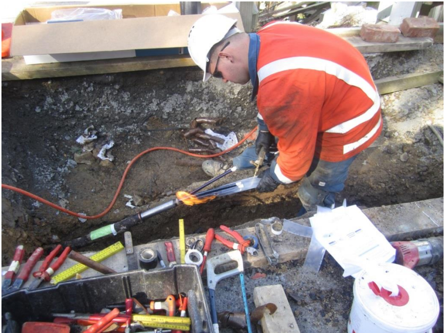
Contractor working on an underground cable
