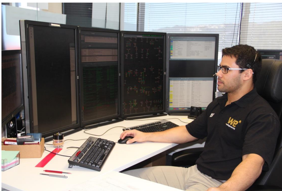
Main Network Control Room
