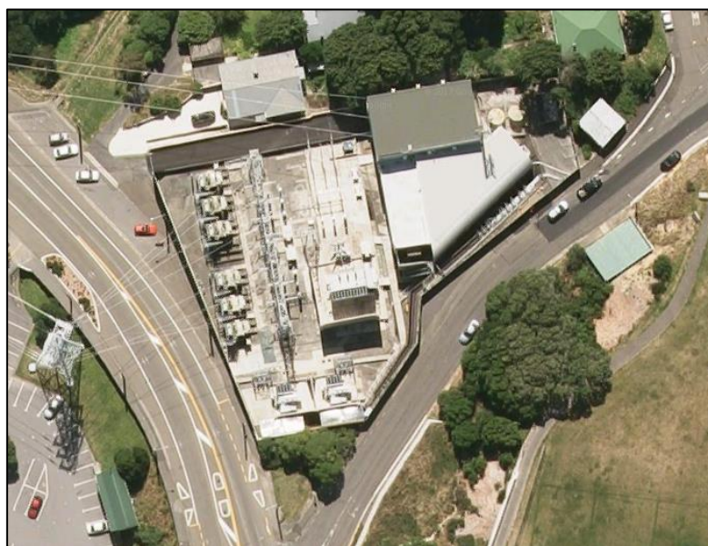
Figure 11-1 Central Park Substation
