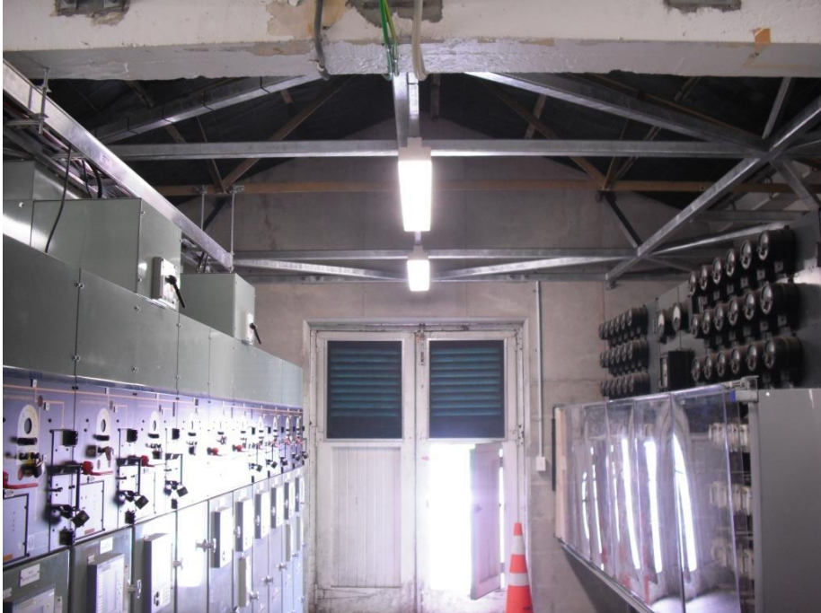
Seismic strengthening at Adelaide Road substation
