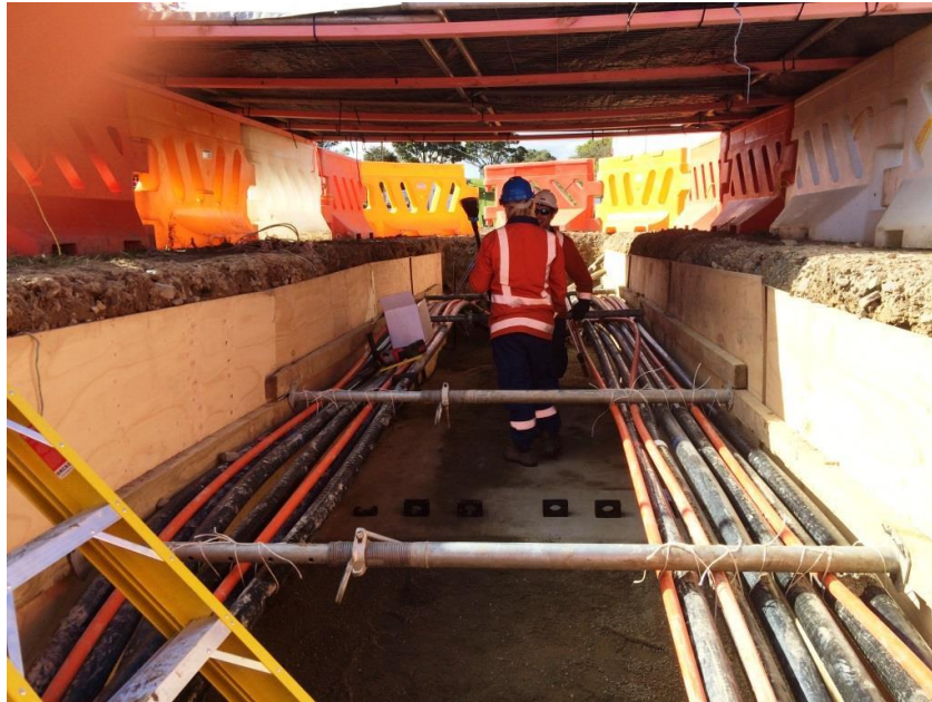
Installation of new 33 kV cables to Palm Grove substation
