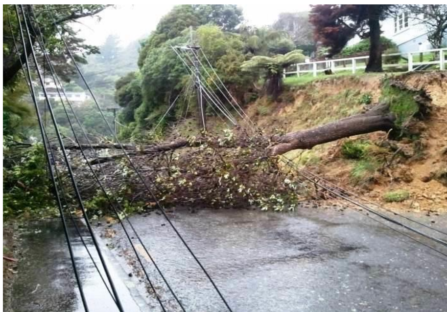
Damage caused during June 2013 storm
