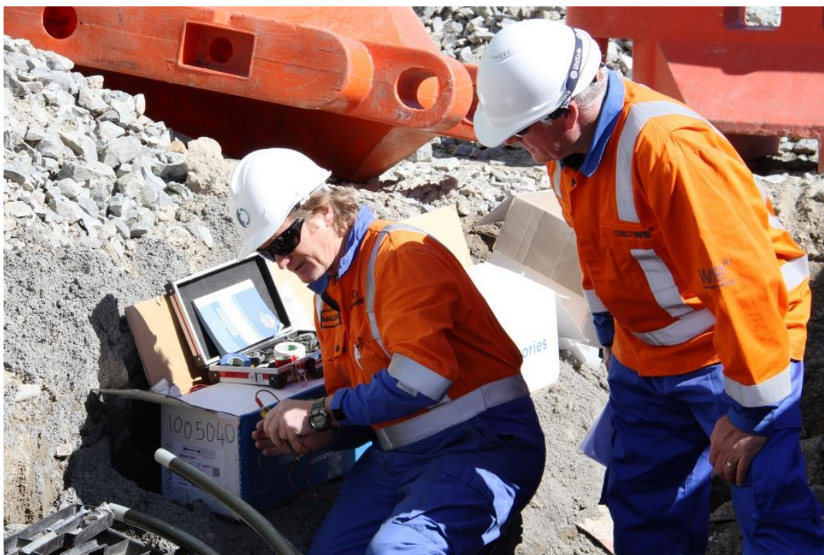
Contractors working on an underground cable
