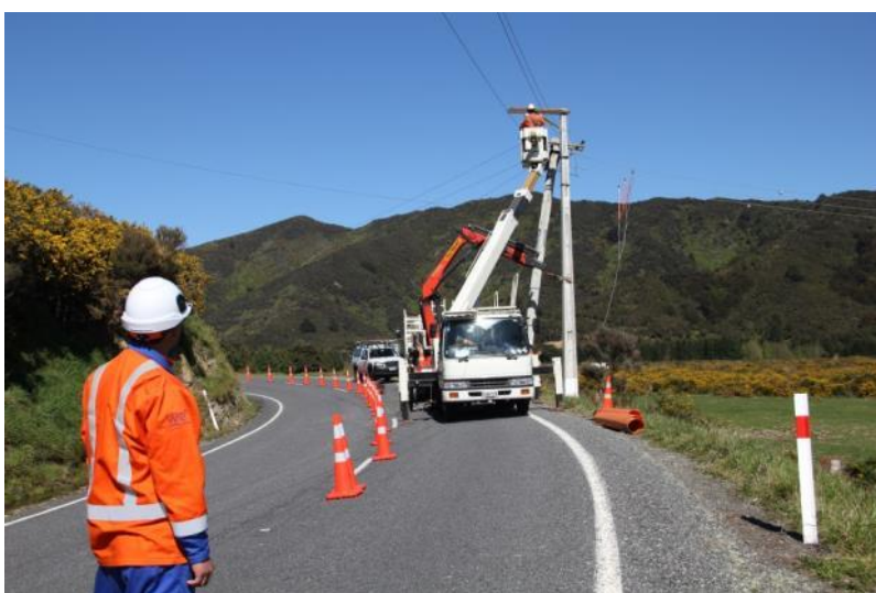
Overhead line refurbishment
