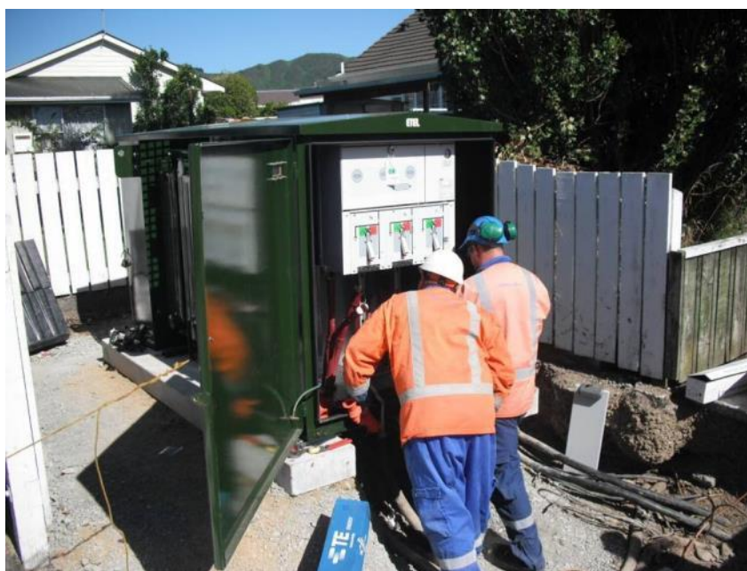
Installation of a replacement distribution substation
