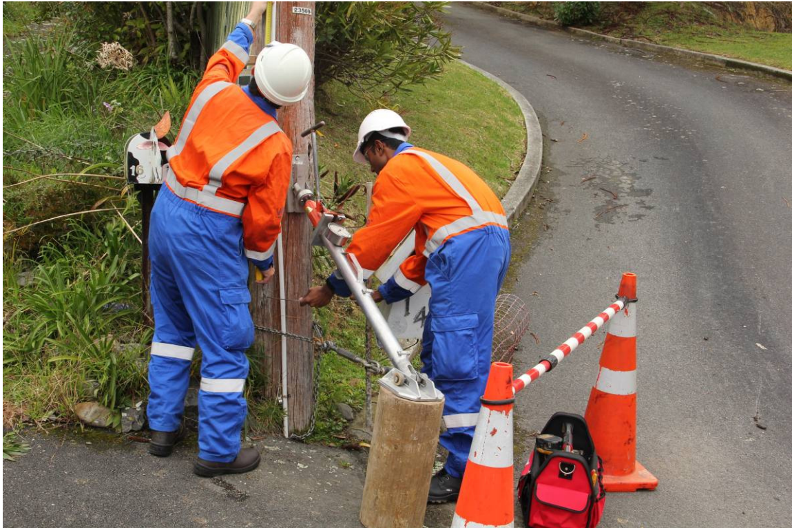
Pole Testing using the Deuar MPT40 test method
