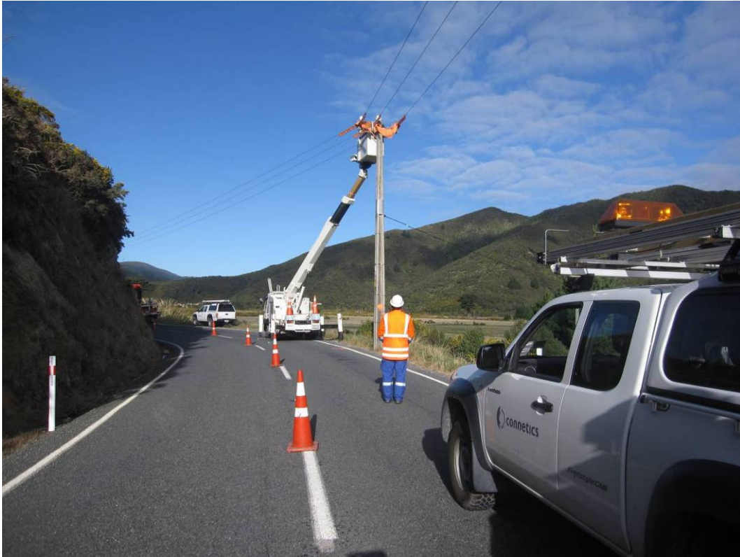
Crossarm replacement in Wainuiomata
