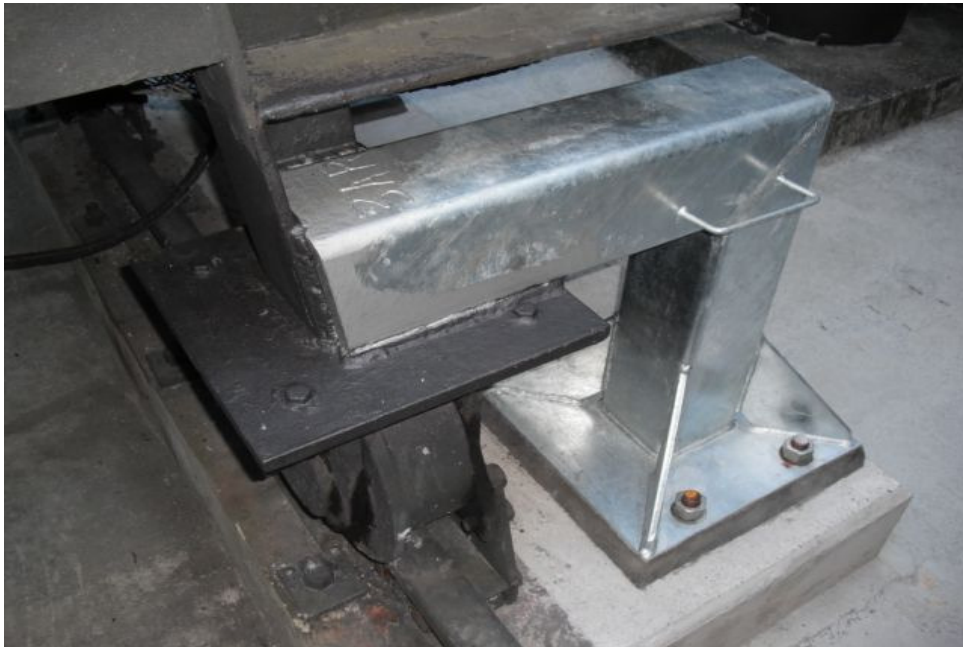
Figure 8-16 Zone Substation Power Transformer Seismic Restraint Footing
