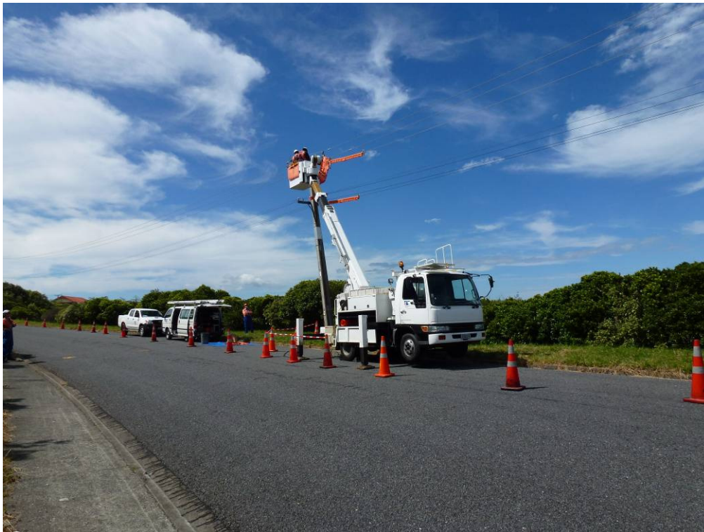
Overhead line work in progress
