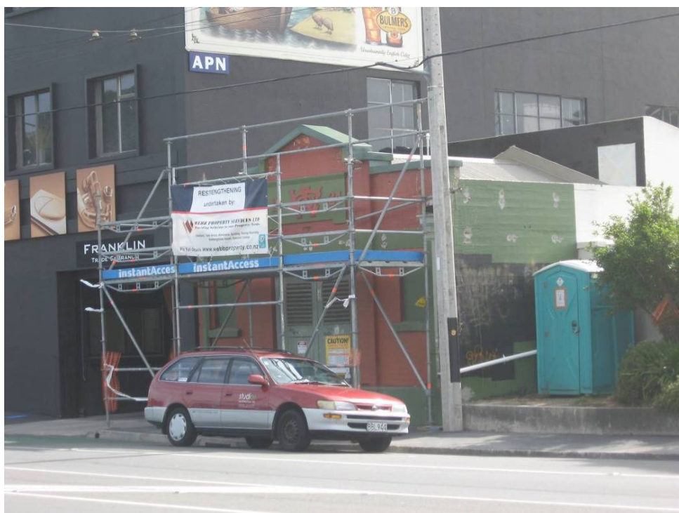
Figure 8-15 Adelaide Road Substation Seismic Reinforcing in progress
