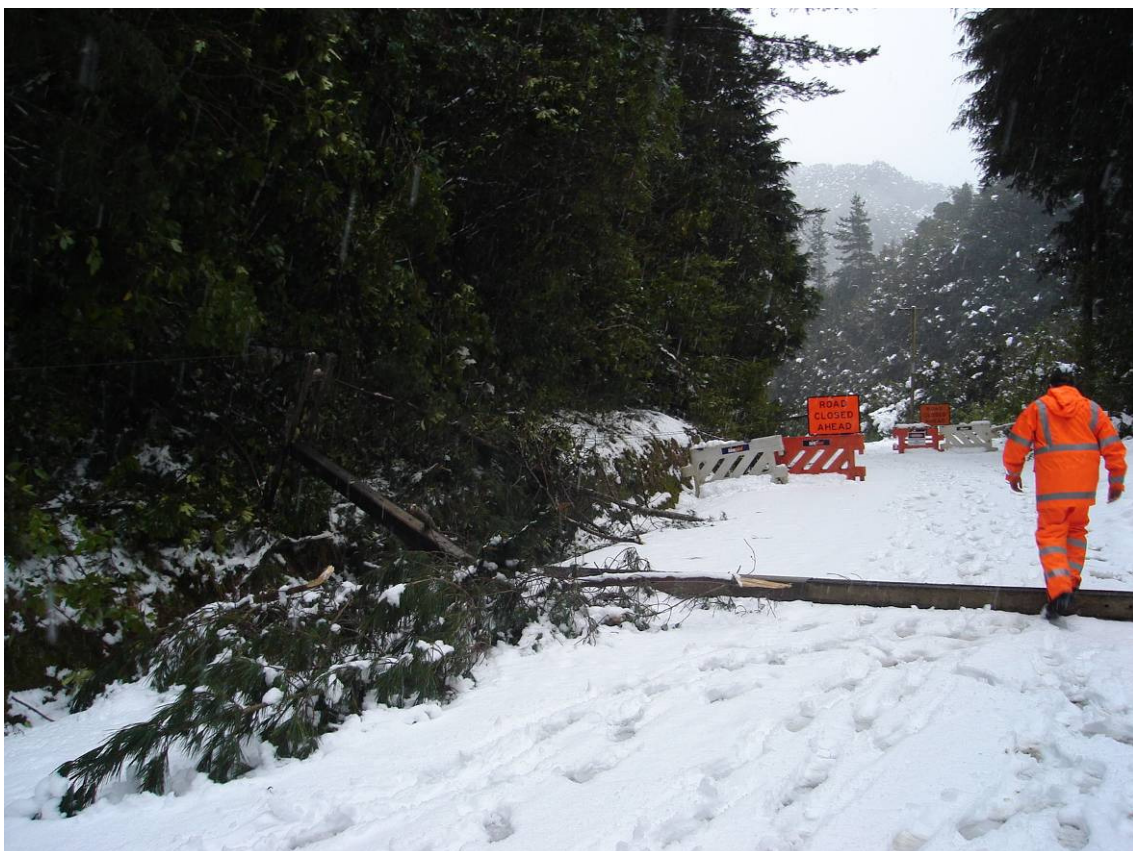
Lines down and broken poles during the August 2011 snow storm
