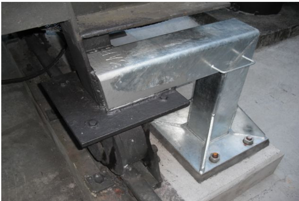
Figure 8-14 Zone Substation Power Transformer Seismic Restraint Footing
