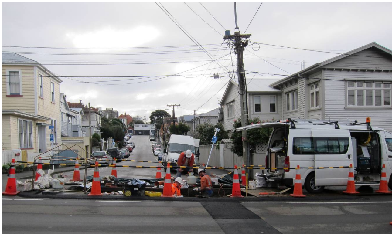
Subtransmission cable jointing in Wellington City
