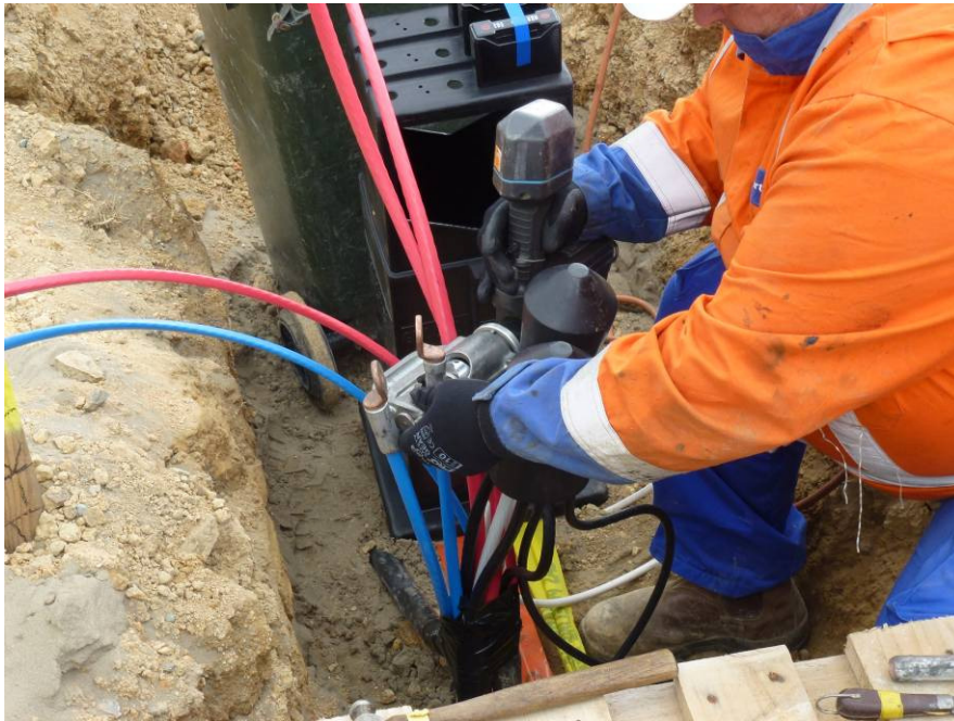
New customer service pillar being installed
