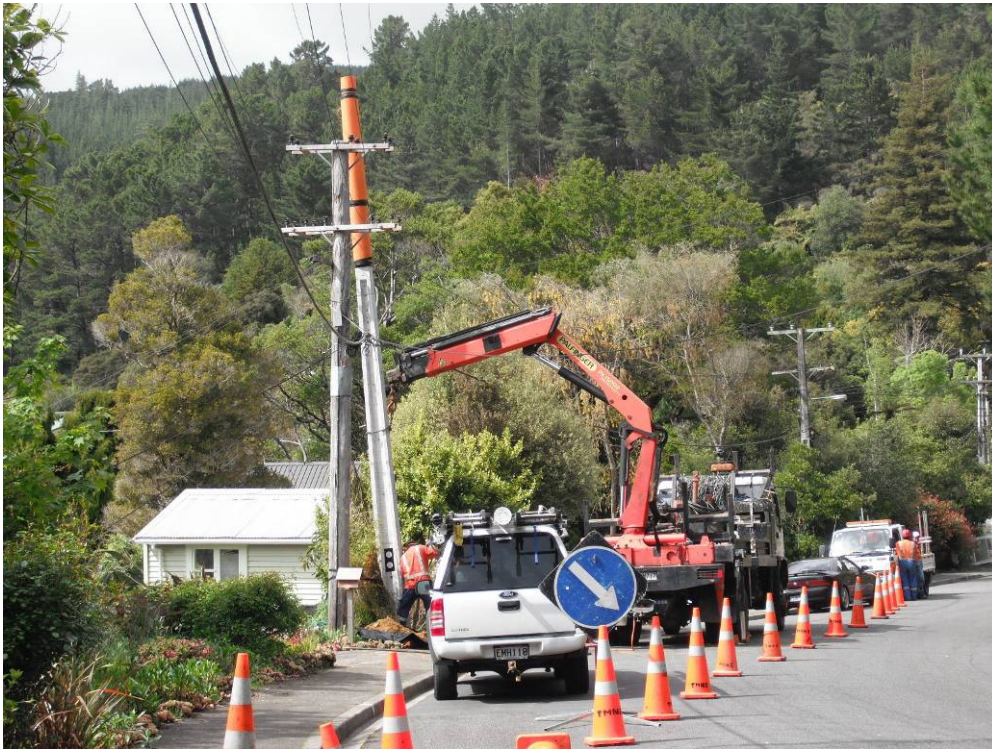
Replacement of an aged timber pole with a new concrete pole
