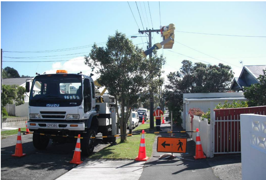
Northpower undertaking overhead network repairs
