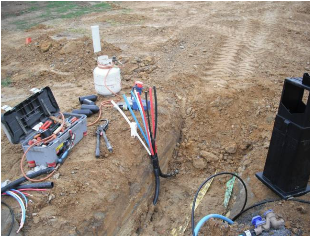
Installation of a new customer service pillar
