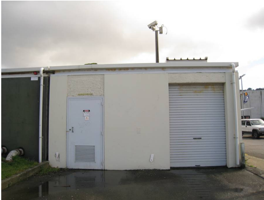
Large distribution substation – concrete block / indoor type
