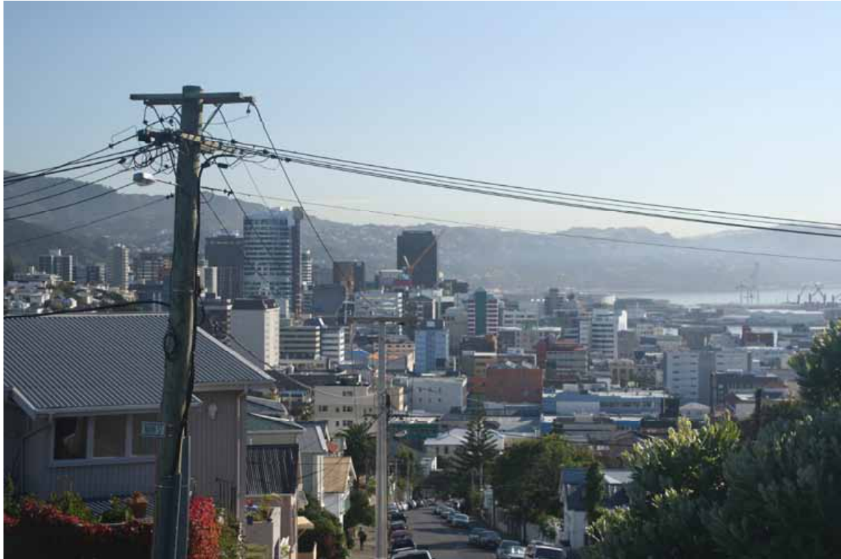
Pole and Overhead Lines – Nairn Street
