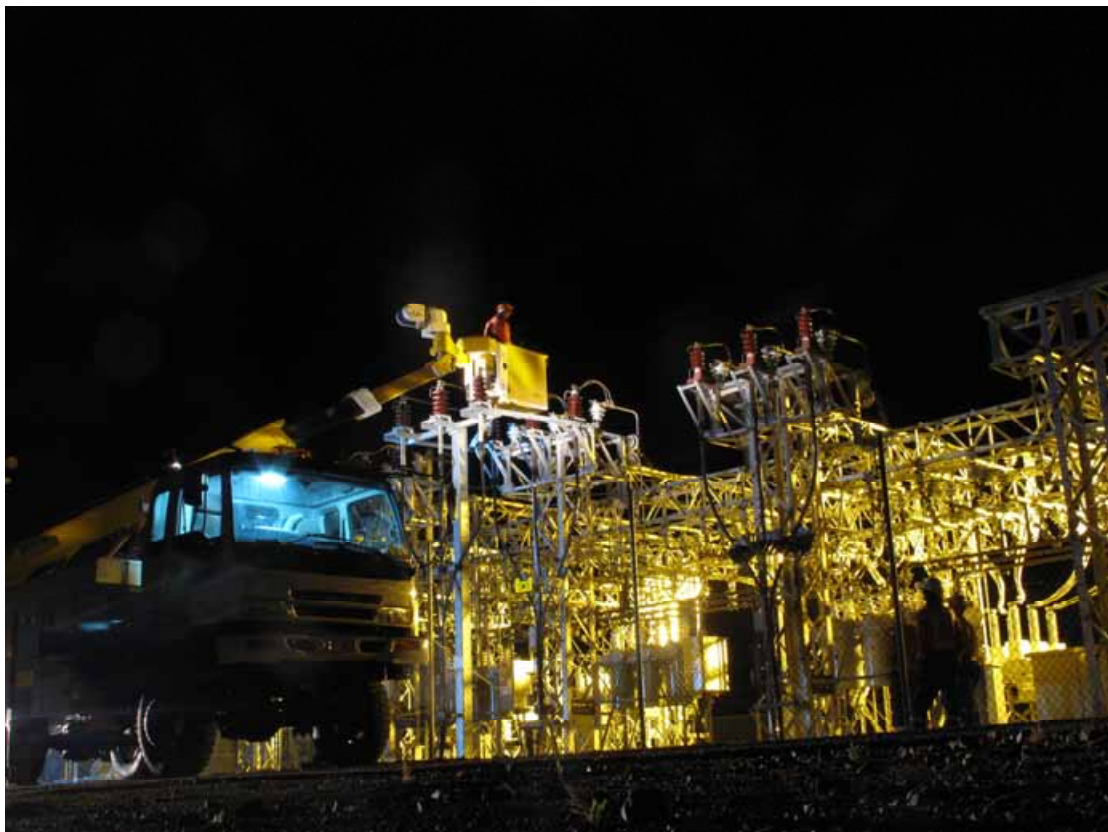
Night Work at Wilton Substation
