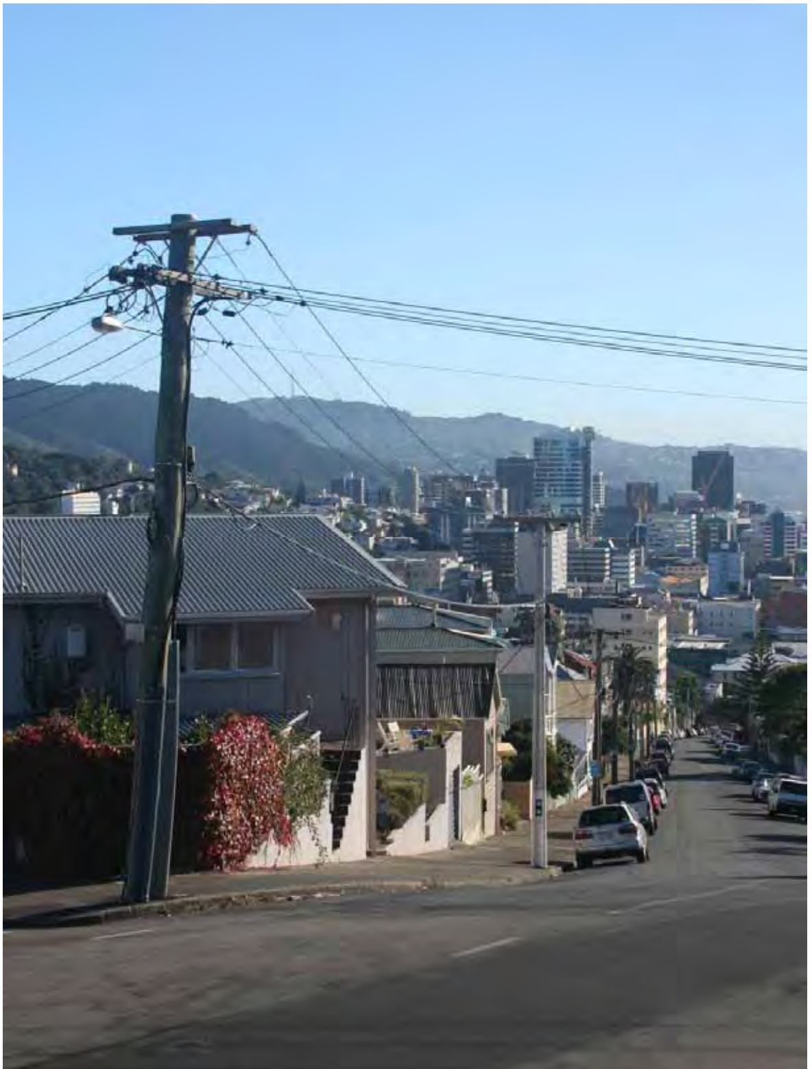
Te Aro Distribution Line
