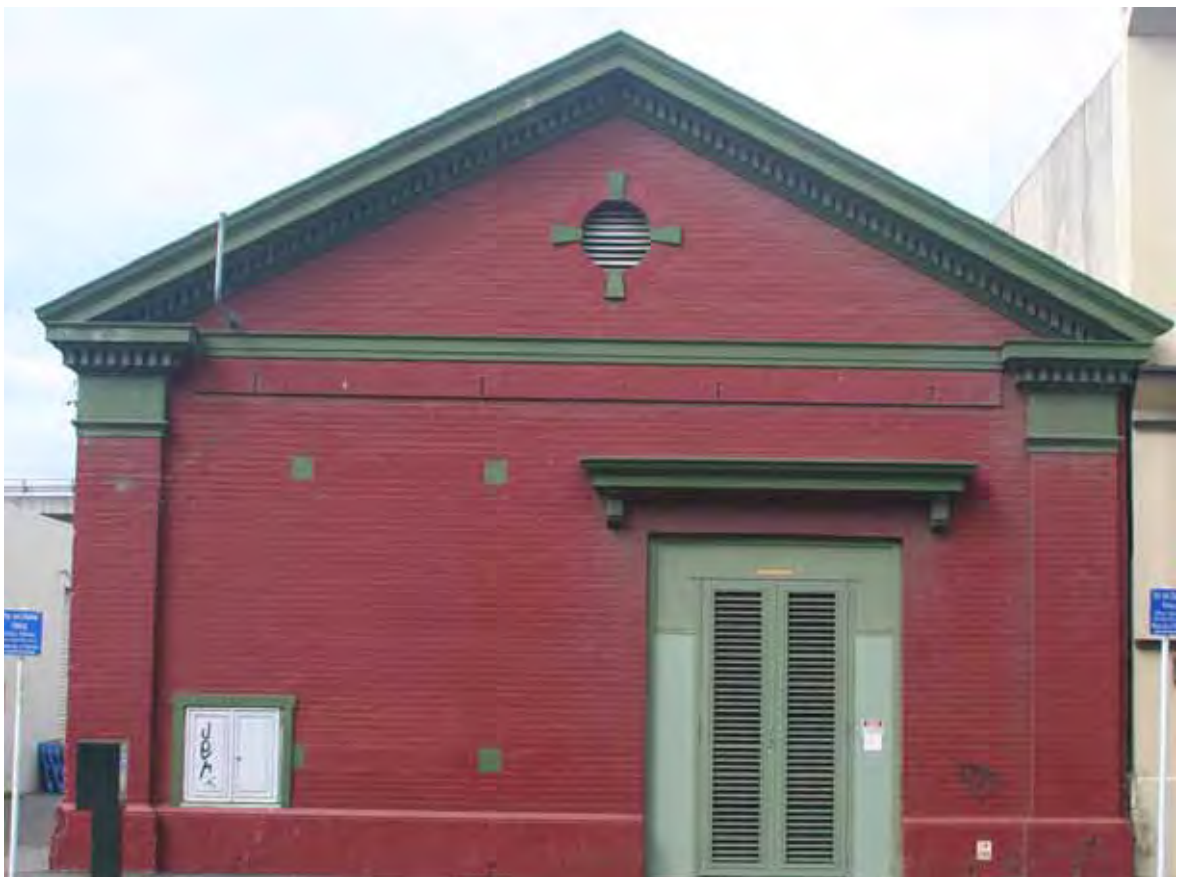
Thorndon Distribution Substation
